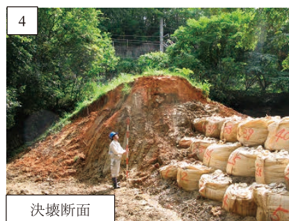
Fig. 9 ②池の決壊断面 Cross section of failure part at ② ike
