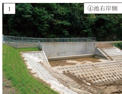
Fig. 16 ④池の洪水吐 Spillway of ④ ike
