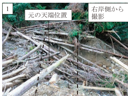
Fig. 21 ⑦池の決壊断面 Cross section of failure part at ⑦ ike
