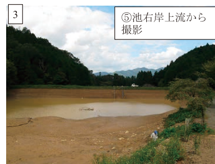
Fig. 18 ⑤池貯水池内の堆砂状況 Sand and mud flowed into ⑤ ike
