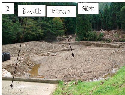
Fig. 13 ③池の貯水池内に流入した土砂 Sand and mud flowed into ③ ike
