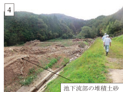
Fig. 24 ⑦池下流部の堆積土砂 Deposited sand at downstream part of ⑦ ike
