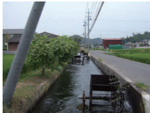
Fig. 58 祐安地区の揚水水車 Irrigation Water Wheel in Sukeyasu district
