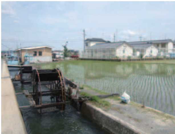
Fig. 39 祐安地区の揚水水車の一例 (木製) Irrigation Water Wheel in Sukeyasu district
