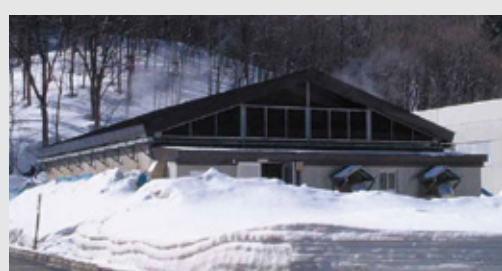
Rock Wool-type Deodorization Facility for Cold Climate
