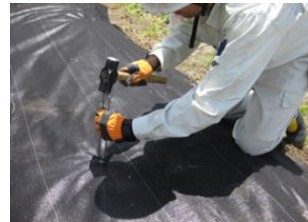
止めピン打設
