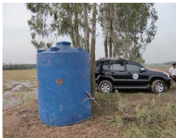
Fig. 8 Storage tank of digested slurry
