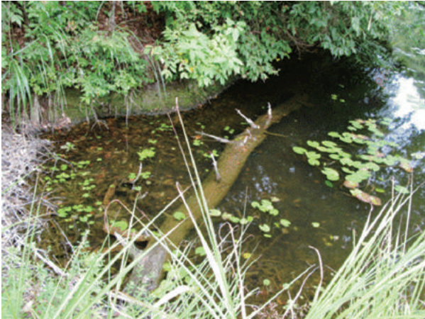
Fig.2-4 洪水吐流入口に漂着した流木 The driftwood which was cast ashore in spillway
